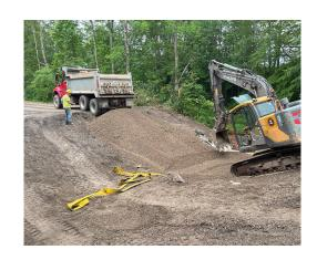
To address the structural and hydraulic challenges of the site, Soleno manufactured and delivered three 20-foot pipes, each with an 84-inch diameter, directly to the project location.
